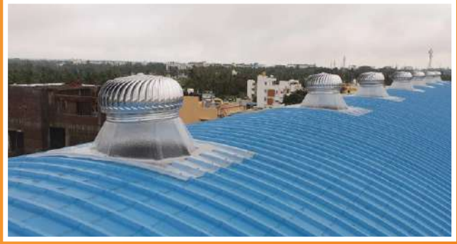
POLYCARBONATE BASE PLATE WITH ALUMINUM VENTILATOR
