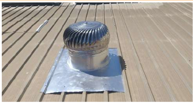
ALUMINUM SIDE END BASE PLATE WITH ALUMINUM VENTILATOR
