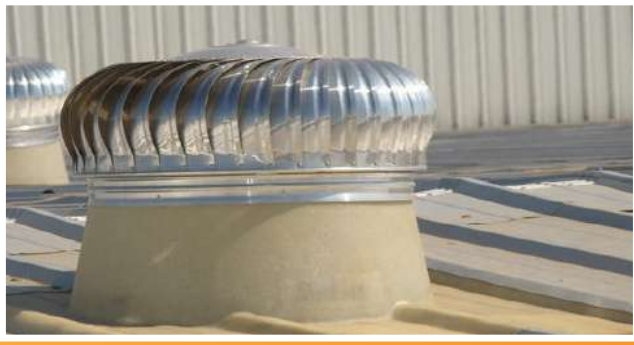
FRP BASE PLATE WITH ALUMINUM VENTILATOR
